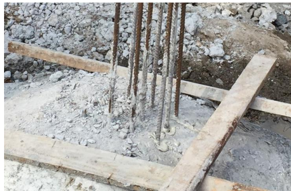
Figure 1. Inappropriate solution for footing location correction. Source: Authors (2016)
