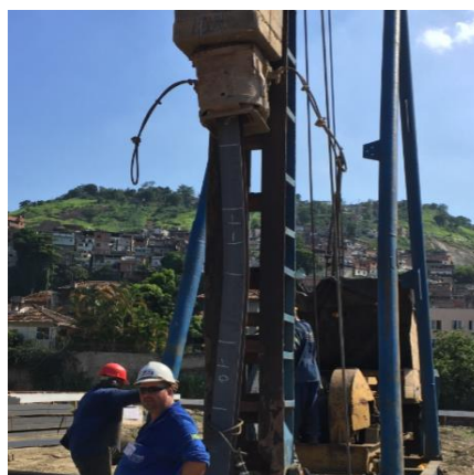
Figure 2. Bucking of a steel pile with W150x37.1. Source: Authors (2016)
